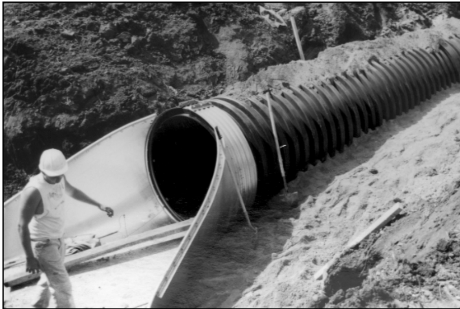
Figure 3-4: Highway Drainage Culvert with HDPE Flared End Section
