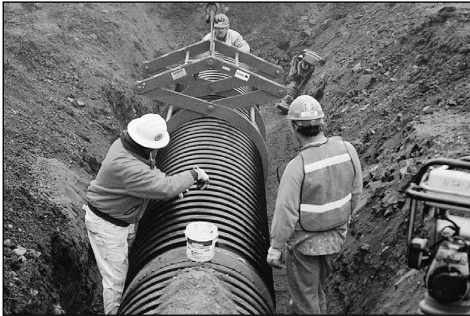
Figure 3-3: Use of a Gasketed Coupling for HDPE Sewer Pipeline Application
